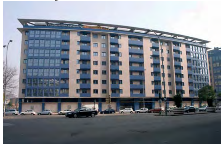
Puerta Real Building, Sevilla
