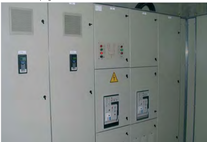
Badalona Pumping Station
