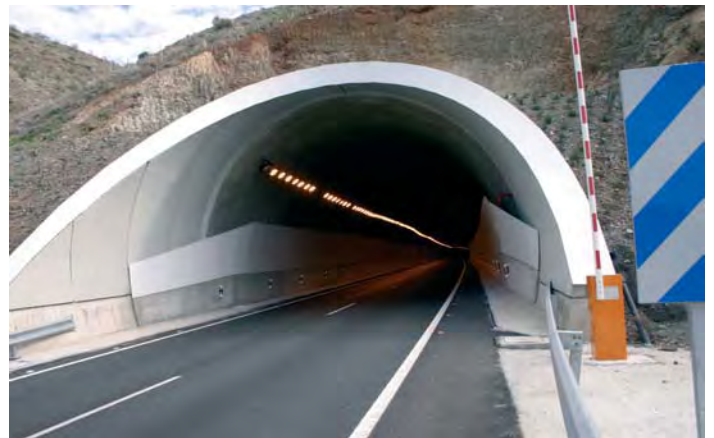
Castel de Ferro tunnels, Granada
