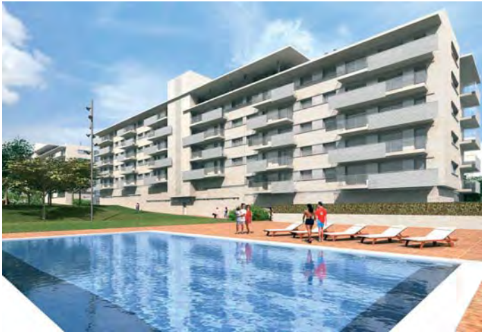
Espai Bulevard Development, Tarragona
