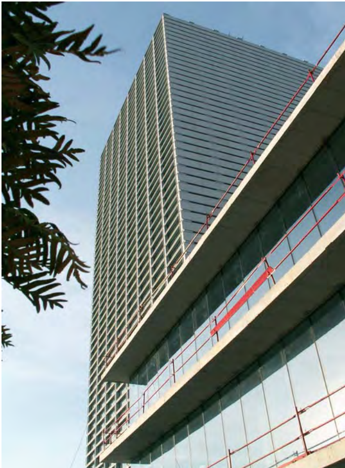
Office building in Boavista Avenue (Porto)
