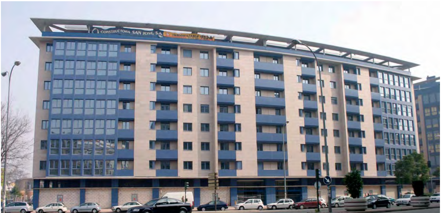
Puerta Real Building, Sevilla.
