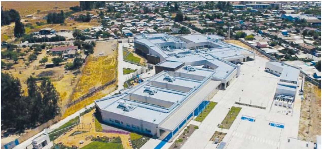
Hospital San José de Casablanca (Chile)
